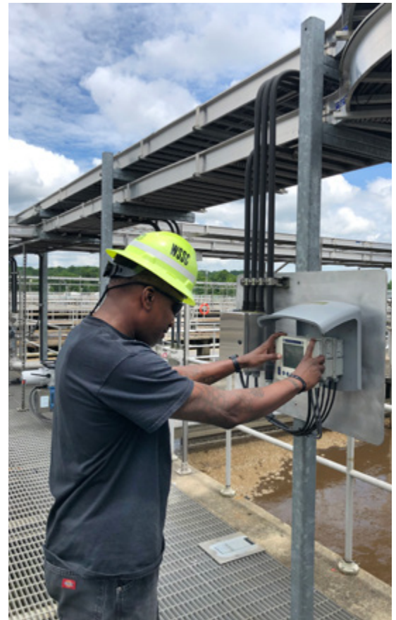
At the Western Branch, Lydell Washington checks real-time nutrient measurements on the IQSN 2020 3G controller.
