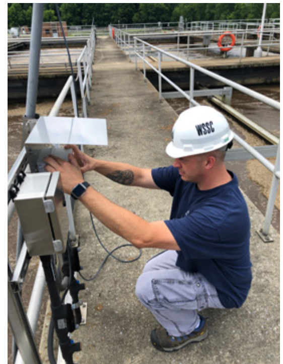
Dave Kramer, Chief Plant Operator for the WSSC Western Branch Facility
